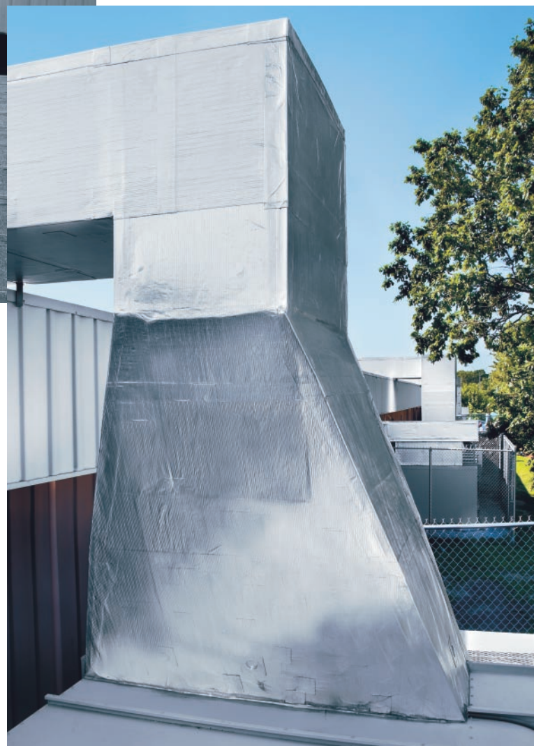
FlexClad-400 can be applied to virtually any shape or configuration. It completely protects the ductwork from infiltration of outside moisture and harmful sunlight, and is warranted by MFM for 10-years.
