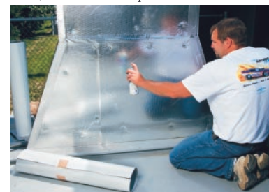
All surfaces should be clean, dry and warm. Use MFM Spray Adhesive to improve adhesion in shaded/shadowed areas, on the bottoms of ducts, and in cool temperatures.
