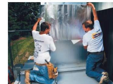
Cut the next section to size overlapping the previous section by at least 3" in order to create a secure, water-resistant seal.
