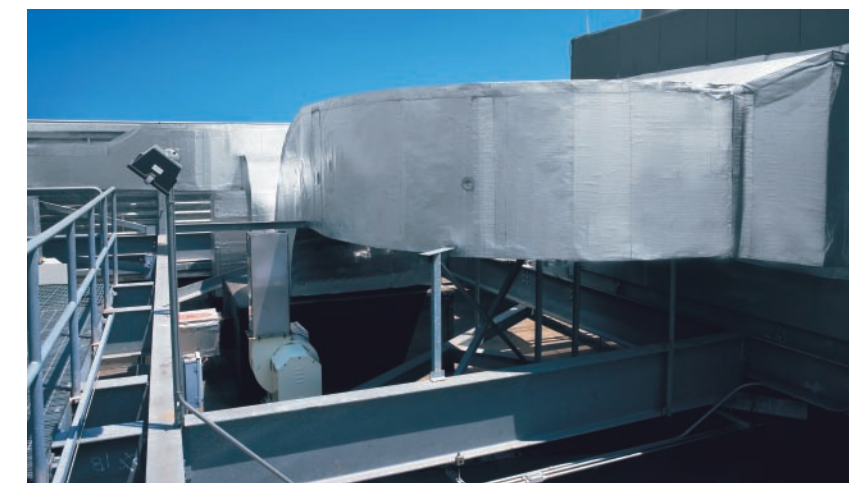
The aluminum top surface is an extremely durable laminated film that is both highly tear- and puncture-resistant. FlexClad-400 is also available in four different color choices in order to allow you to blend your system to the surrounding structure.
