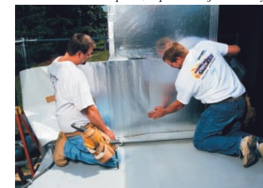
After measuring and cutting the section to the proper size, align and gently press FlexClad-400 into place; reposition if necessary.
