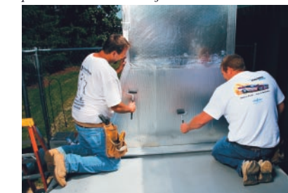
Complete the installation by applying firm pressure to the entire surface with a hand roller.
