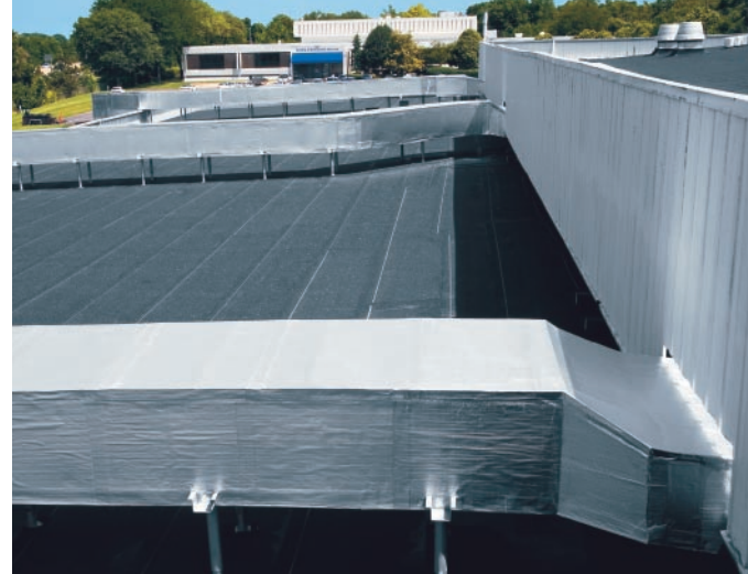
For straight, long length duct systems, FlexClad-400 makes for a clean, uncluttered appearance. Quickly and easily installed, it replaces expensive and cumbersome metal jacketing commonly used to protect insulated ductwork.
