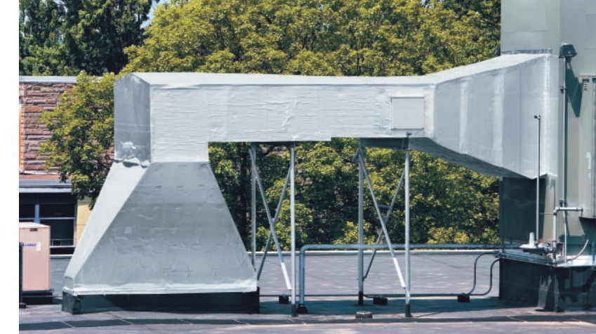
Unlike competitor products, the 40 mil thickness of FlexClad-400 provides excellent weather and self-sealing protection without the excess weight of unnecessary "filler" materials in its composition.
