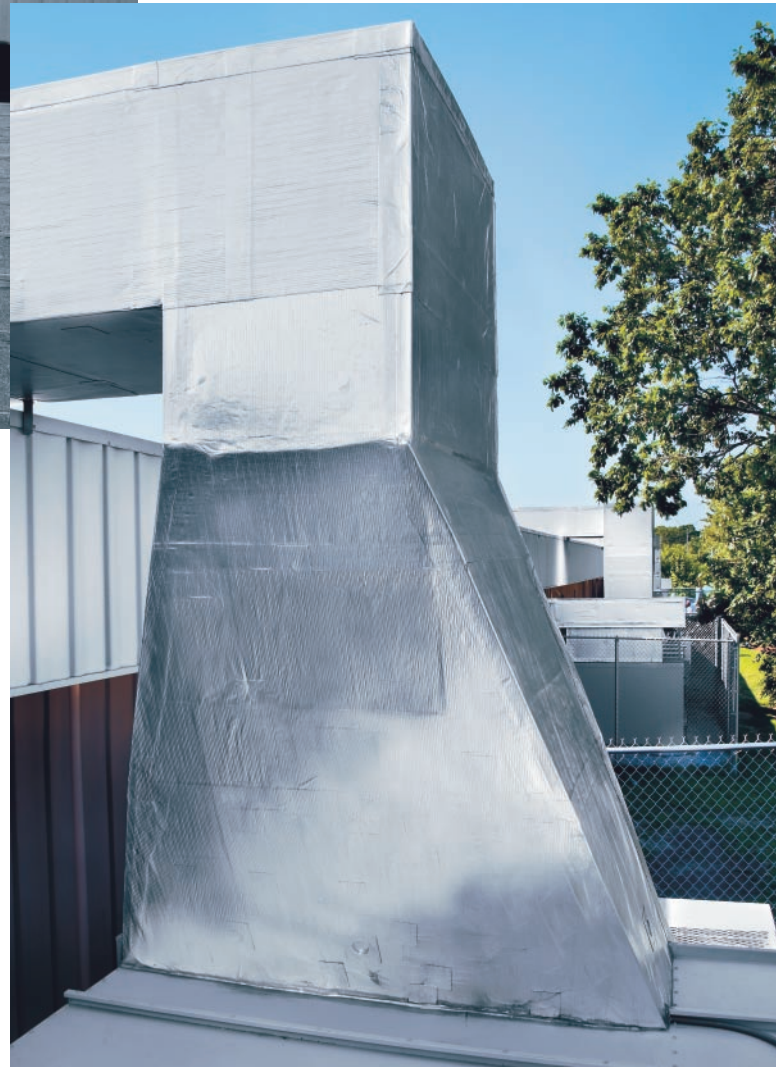
FlexClad-400 can be applied to virtually any shape or configuration. It completely protects the ductwork from infiltration of outside moisture and harmful sunlight, and is warranted by MFM for 10-years.
