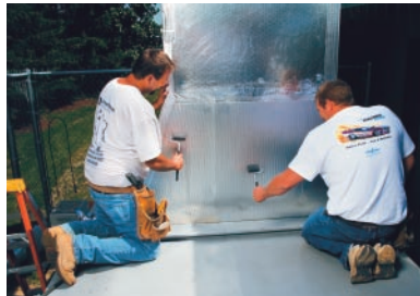
Complete the installation by applying firm pressure to the entire surface with a hand roller.
