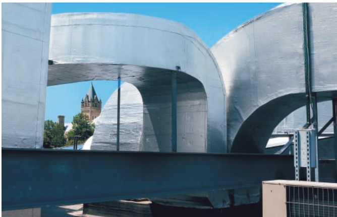
Potentially difficult installations that include sweeping curved corners and odd shapes are made easy with FlexClad-400, and its excellent elongation characteristics accommodate structural movement.
