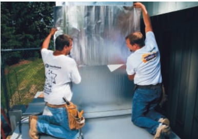
Cut the next section to size overlapping the previous section by at least 3" in order to create a secure, water-resistant seal.
