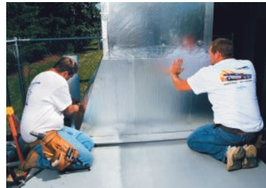
When in final position, firmly hand seal to the surface and fold over all edges as shown.
