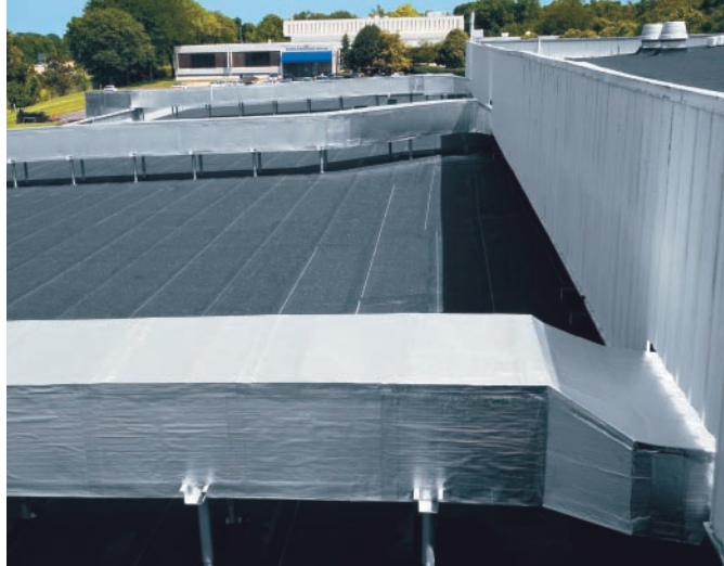
For straight, long length duct systems, FlexClad-400 makes for a clean, uncluttered appearance. Quickly and easily installed, it replaces expensive and cumbersome metal jacking commonly used to protect insulated ductwork.
